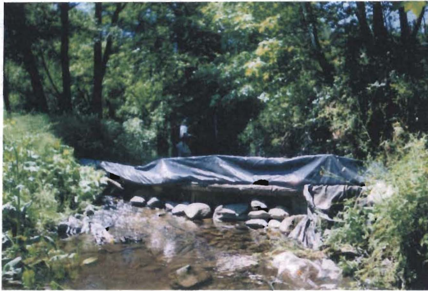
Figure 3.10 – Channel spanning push up dam in Thompson Creek
